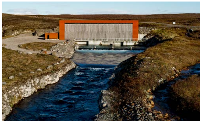
HS Orka's electricity generation portfolio includes two hydropower facilities
